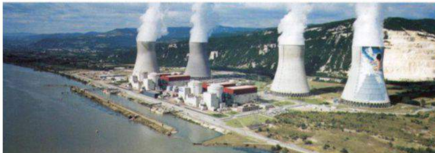
The four PWR units of Cruas, France with seismic isolation
